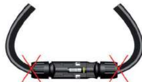
Incorrect routing of cable
