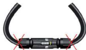
Incorrect routing of cable
